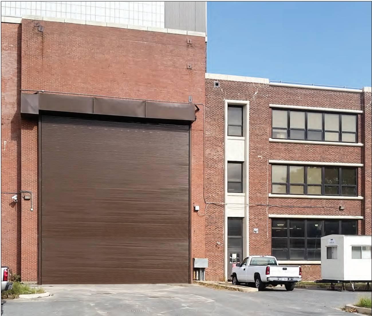
Fully operational while subjected to a sustained 110 mph wind load – with no damage or deformation.
